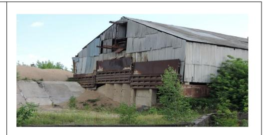
Aggregate unloading complex with a three-hopper device
